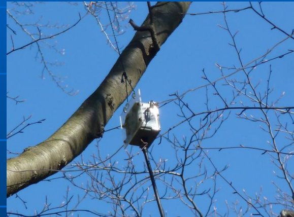
80M Off Center Fed Dipole (Works on 80, 40, 30, 20, 17,24,28,54 MHz Bands)
